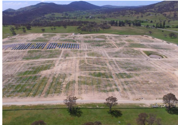
Williamsdale Solar Farm – built by Director Glenn Melton between Canberra and Cooma. Is 11.87MW in size on Single Axis Tracking with Central Inverters.
