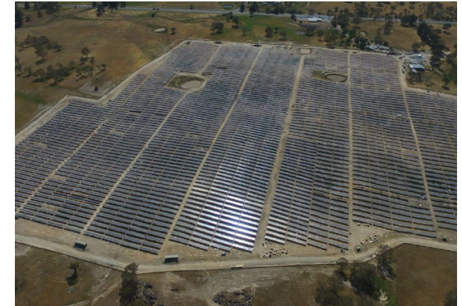
Williamsdale Solar Farm – built by Director Glenn Melton between Canberra and Cooma. Is 11.87MW in size on Single Axis Tracking with Central Inverters.
